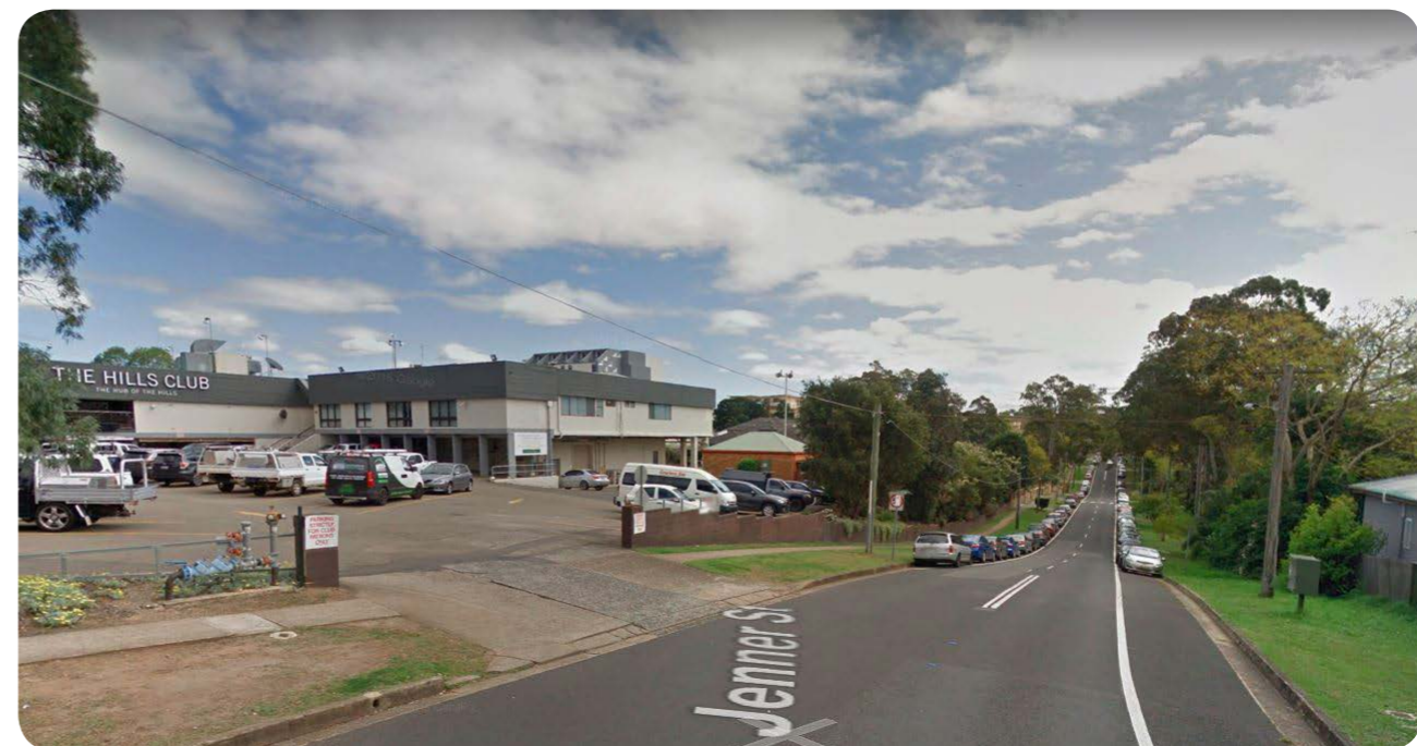
4. VIEW OF SITE FROM JENNER STREET HEADING NORTH
